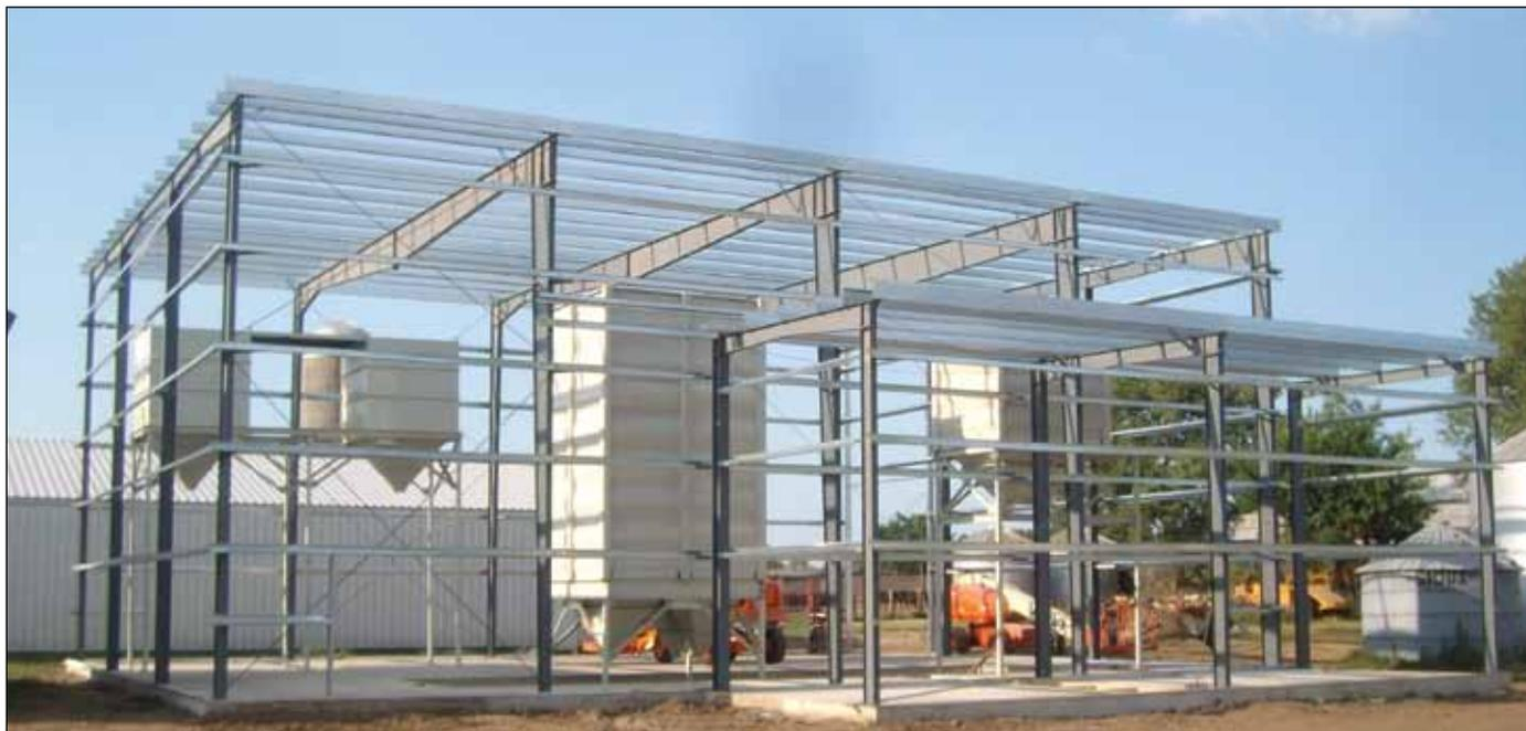
Steel framework of Epley Brothers Hybrids' 6,000 sq. ft. clear-span conditioning building with receiving annex. Surge bins and bulk storage bins have been installed ahead of conditioning equipment installation. (August 2012 Popp Engineering photo).
